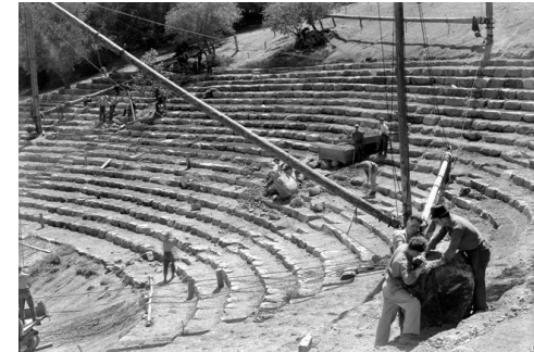
CCC working on the Mountain Theater, 1933
