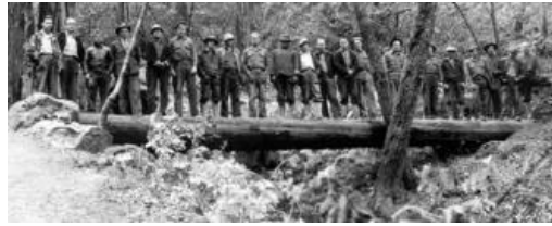
CCC on log bridge project on Ben Johnson Trail
